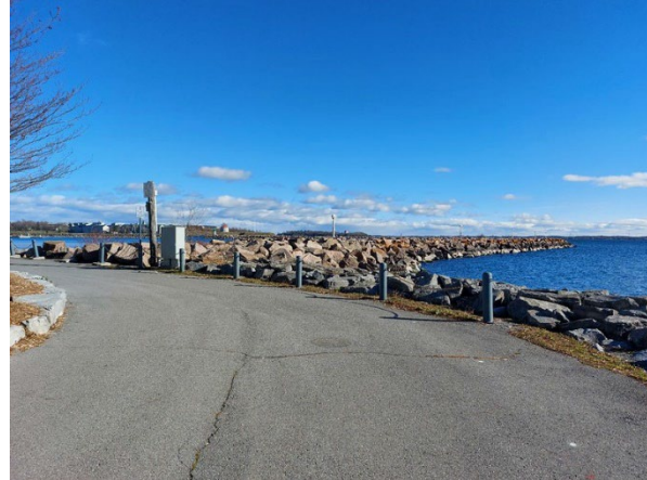
Figure 3. The breakwall, on the Kingston Waterfront GeoWalk.
